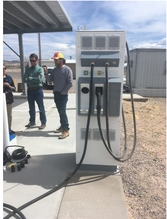
Photo (Above): Dave Luttrell (Lincoln County Power District) explains the DC-FC project to GOE and U.S. DOE staff as they make a site visit to the EV charging station in Panaca, NV. (source: GOE).
